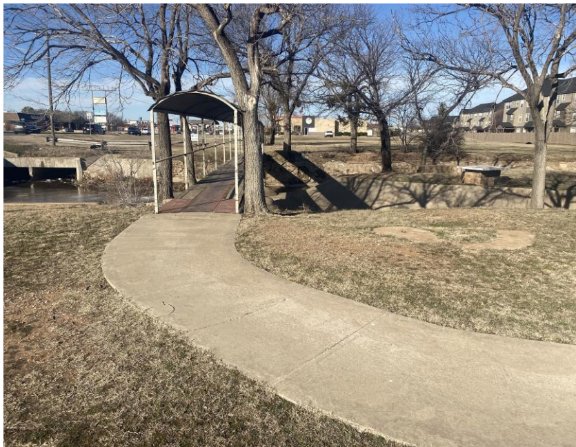
Bridges along a multi-use trail facility at Bridge Park
